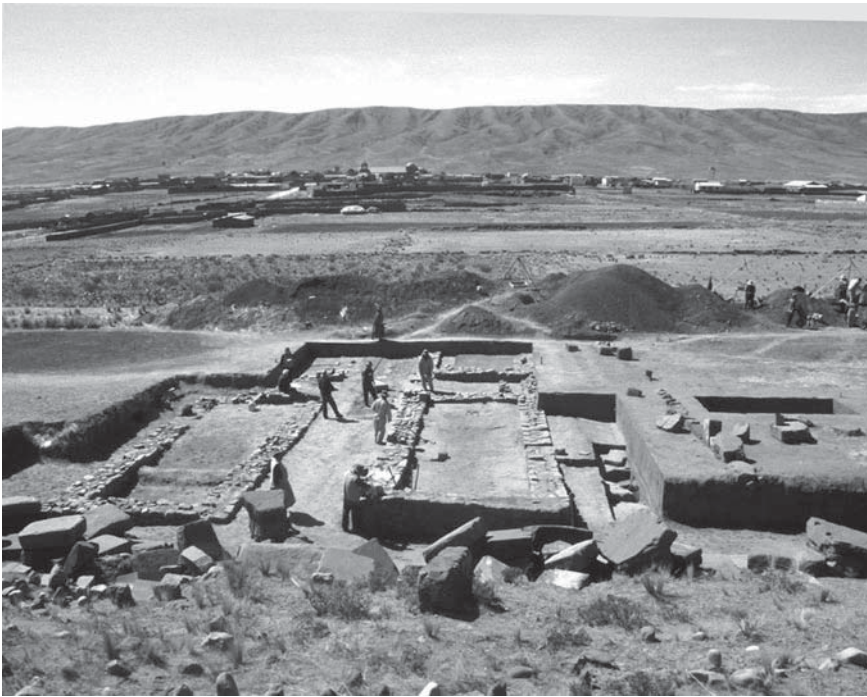
Figura 6: Excavaciones en la zona norcentral de Pumapunku . Excavations in the north-central zone of the Pumapunku.
